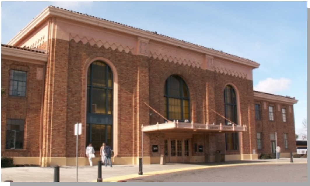
SAN JOSE DEPOT TODAY -- A major renovation in the 1990s of the former Southern Pacific San Jose Depot today provides local and intercity travelers with a fine transportation hub, always ready to offer rail, bus, and light rail transportation services for Santa Clara Valley residents. At 70 years of age, the depot looks ready for another 70 years of service.
